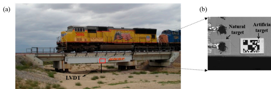
Figure 11. Field test of a railway bridge: (a) Displacement measurement under moving trainloads; (b) Artificial target and natural target.
