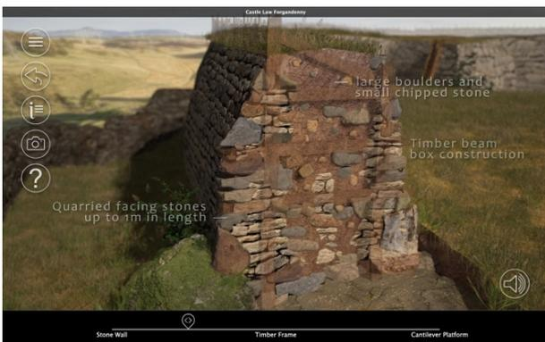
Figure 2: The cut-away reconstruction of the wall at Castle Law Forgandenny.
