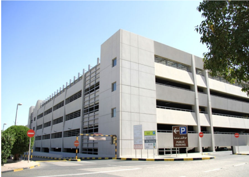
Car Park Before Construction of FICU.
