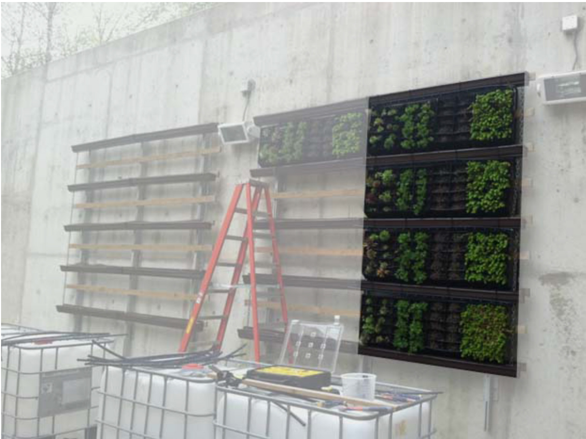
FIGURE 4. Complete greenwall system on the right with start of second system to left.
