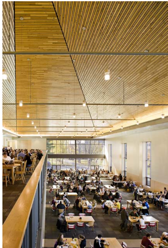
FIGURE 9. High ceilings in the Dining Room help exhaust heat in the summer. The ceilings are made from wood reclaimed from an old Thomas Edison Plant in Wisconsin. Photo: ©Robert Benson.
