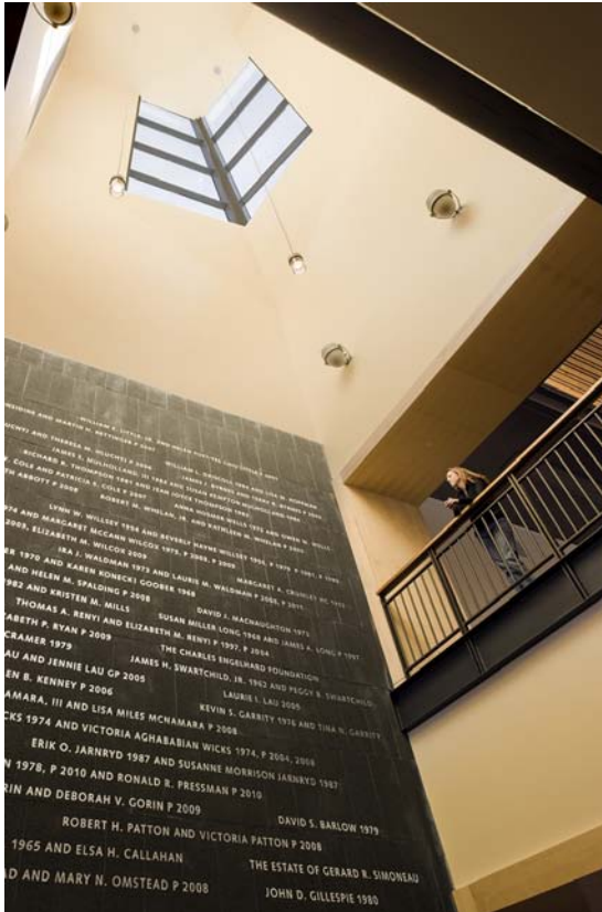
FIGURE 10. The Roof Monitor brings daylight further into the building. A fan at its top exhausts warm air in the summer and recovers heat in the winter. Photo: ©Robert Benson Photography.
