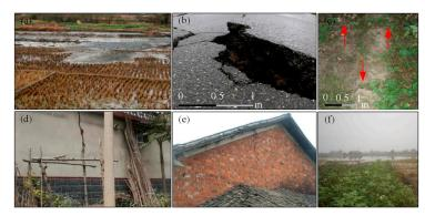
**Figure 4.** In situ pictures of ground ruptures in the rock salt mine. (a) The underground brine flowing into the cultivated land, inducing land salinization. (**b**,**c**) Accumulated deformation induced road surface cracks. (**d**,**e**) Cracks on resident houses (**f**) Gradually formed stagnant water area, with a settlement even deeper than 1.5 m.
