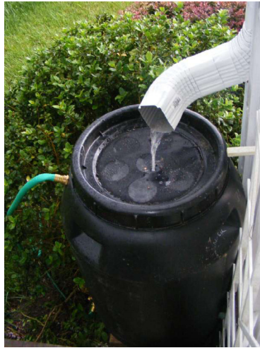
FIGURE 7. A rain barrel system for rain water harvesting. (Photo courtesy Vision Design Collaborative)
