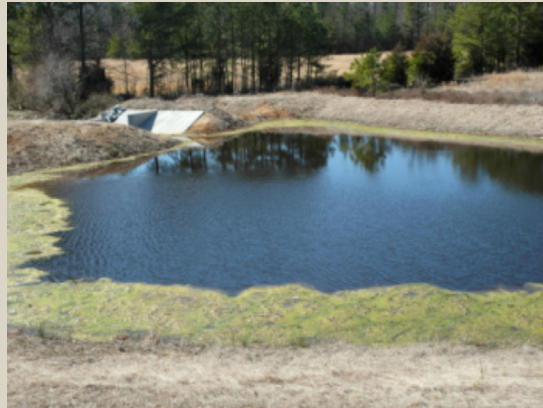
FIGURE 3. A detention pond for stormwater runoff from a new commercial development. (Photo courtesy Stephen Mosberg)
