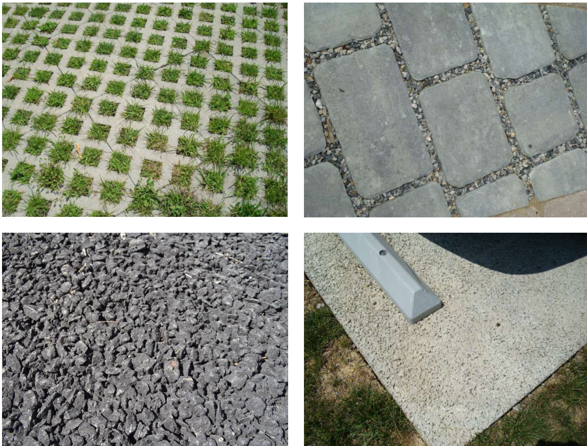
FIGURE 4. Examples of permeable pavement applications: grid pavers; pavers; permeable asphalt; and permeable concrete. (Images courtesy Laurie Fox)
