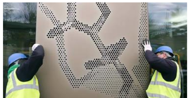
Figure 3: The Panels being installed
