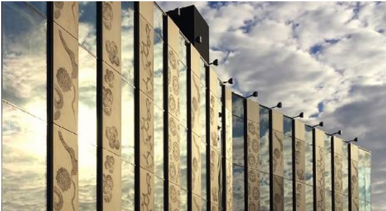
Figure 4: The panels installed on the north side of the building
