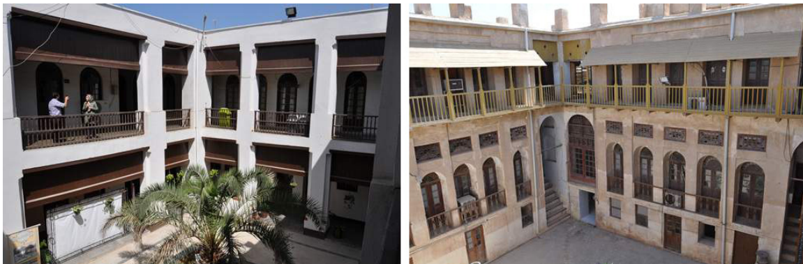
FIGURE 13. Porous facades and large openings in tropical region of Persian Gulf. The openings facilitate natural ventilation (courtesy of Sara Fadaei Nejad).
