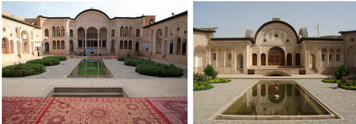
FIGURE 8. Differences of size of openings between southern façade and northern façade in a courtyard house in hot arid climate of Iran (courtesy of authors).
